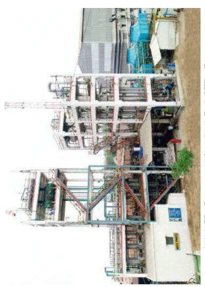
Multiple Effect Evaporator with Crystallizer in Textile CETP at Tiruppur
